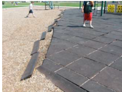
Dual surface failure
