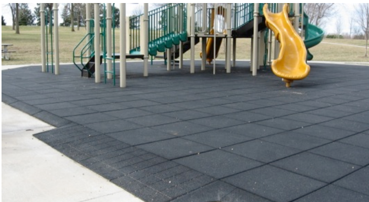
Bevel ramp from access route
